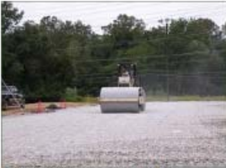
4. Placement of open-graded aggregate base stone.
