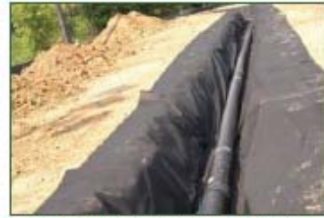
3. Installation of underdrain piping system and geo-textile fabric.
