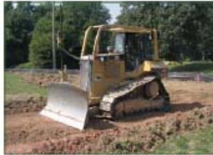
2. Stripping vegetation and topsoil from existing rectangular field.
