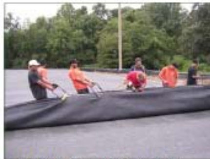
5. Synthetic turf installation. Turf is secured and sewn.
